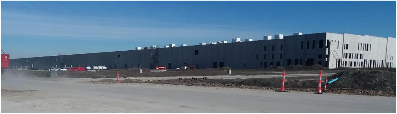
World Wide Technology Building 2 – Edwardsville, Illinois
