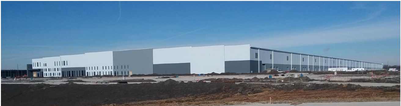
World Wide Technology Building 1 – Edwardsville, Illinois
